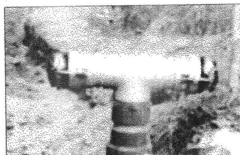
Fig: QRC outlet, easy to connect with other pipes
