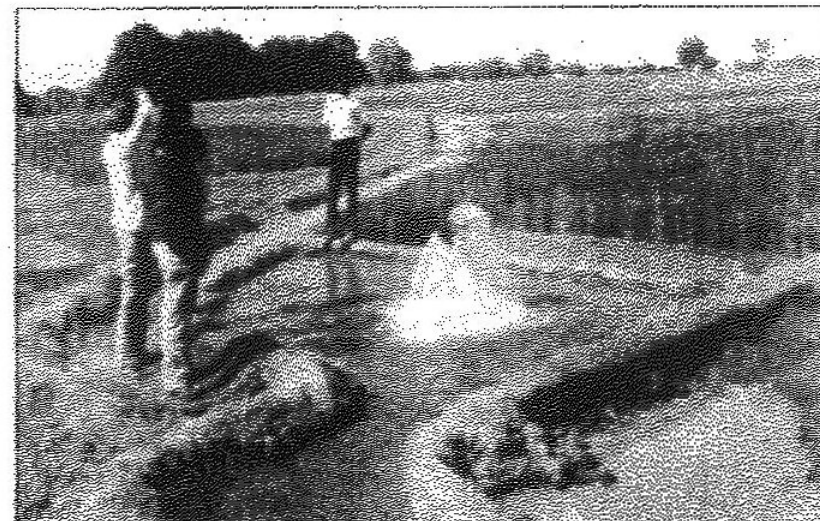
Fig: Water coming out of an outlet of micro LI system
